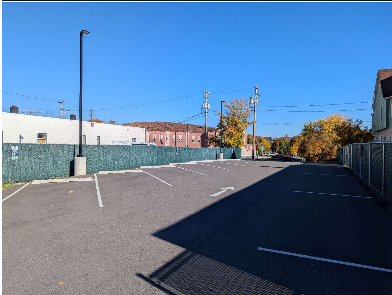
Figure 7: No Lighting Elements Along Eastern Perimeter of Main Street Lot (October 2024)
