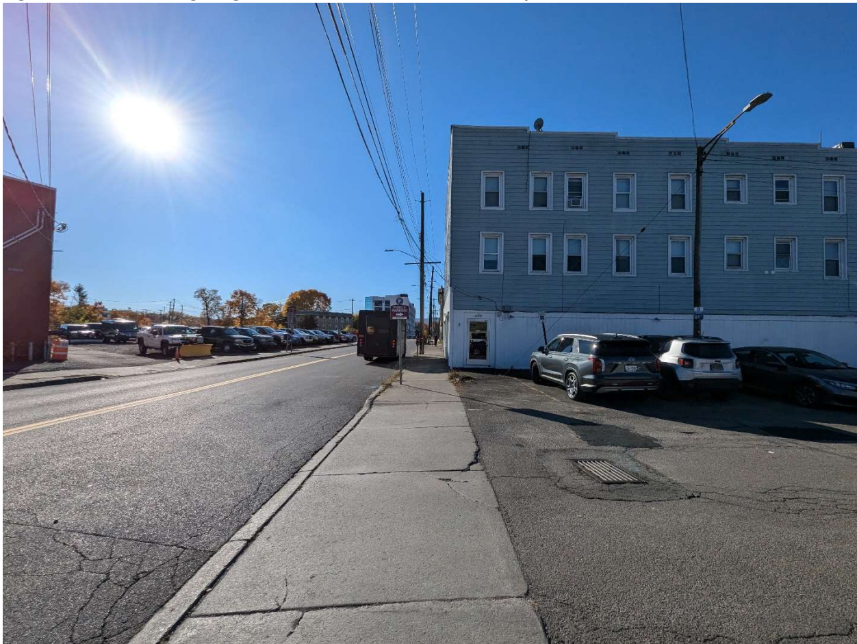
Figure 5: Absence of Lighting Elements over Willow Street Entry/Exit for Willow Lot (October 2024)
