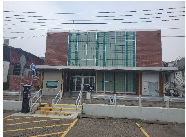
Rear of Old Village Hall.
